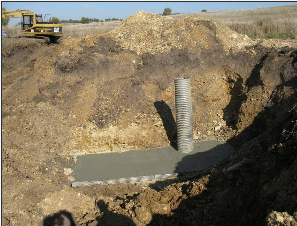
High strength concrete was poured over the works.
