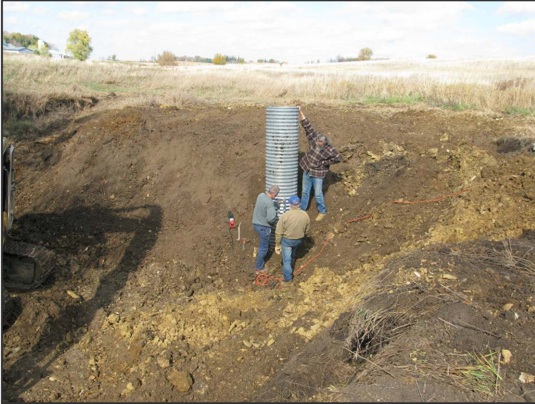
The site was partially backfilled and a culvert extension was added.
