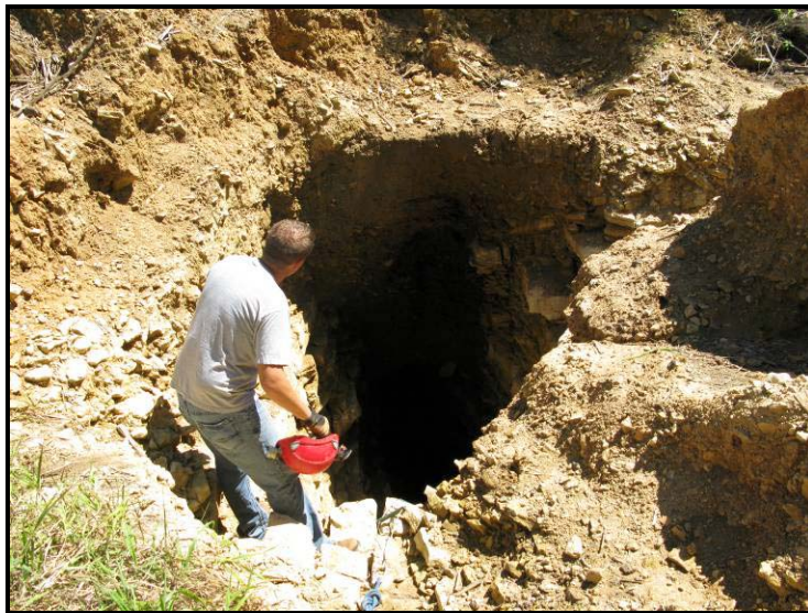
Dan Dornink inspects the newly opened gaping hole.
